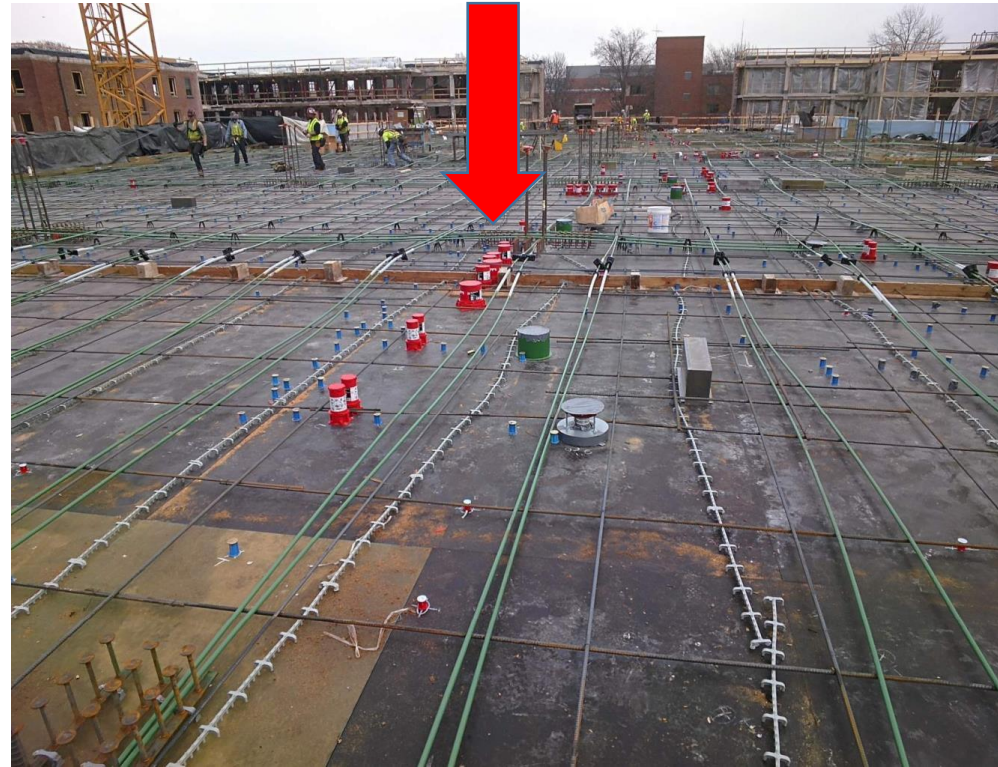
PT Cabling, M & E Sleeves
