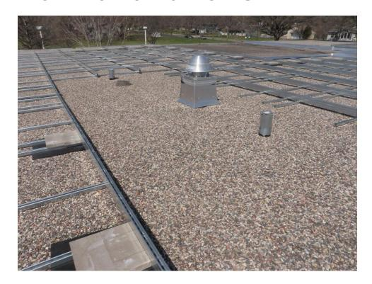
Ensure Roof Membrane Protected From Damage During Install
