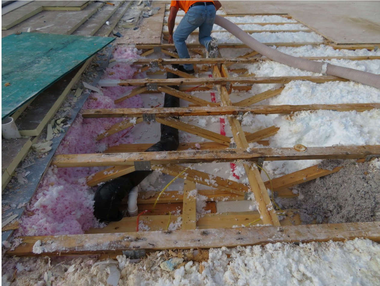
Blown-in insulation
