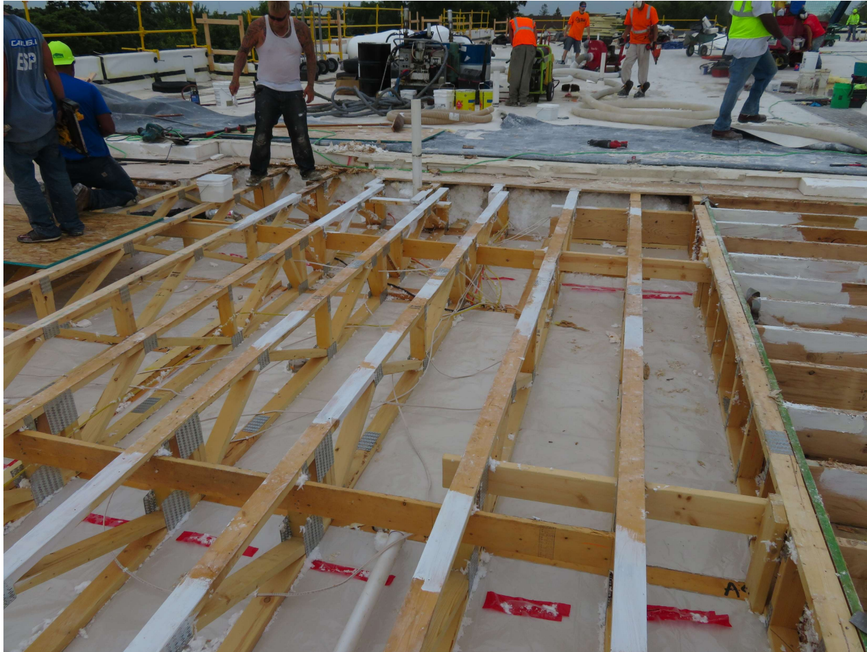
Mold remediation paint
