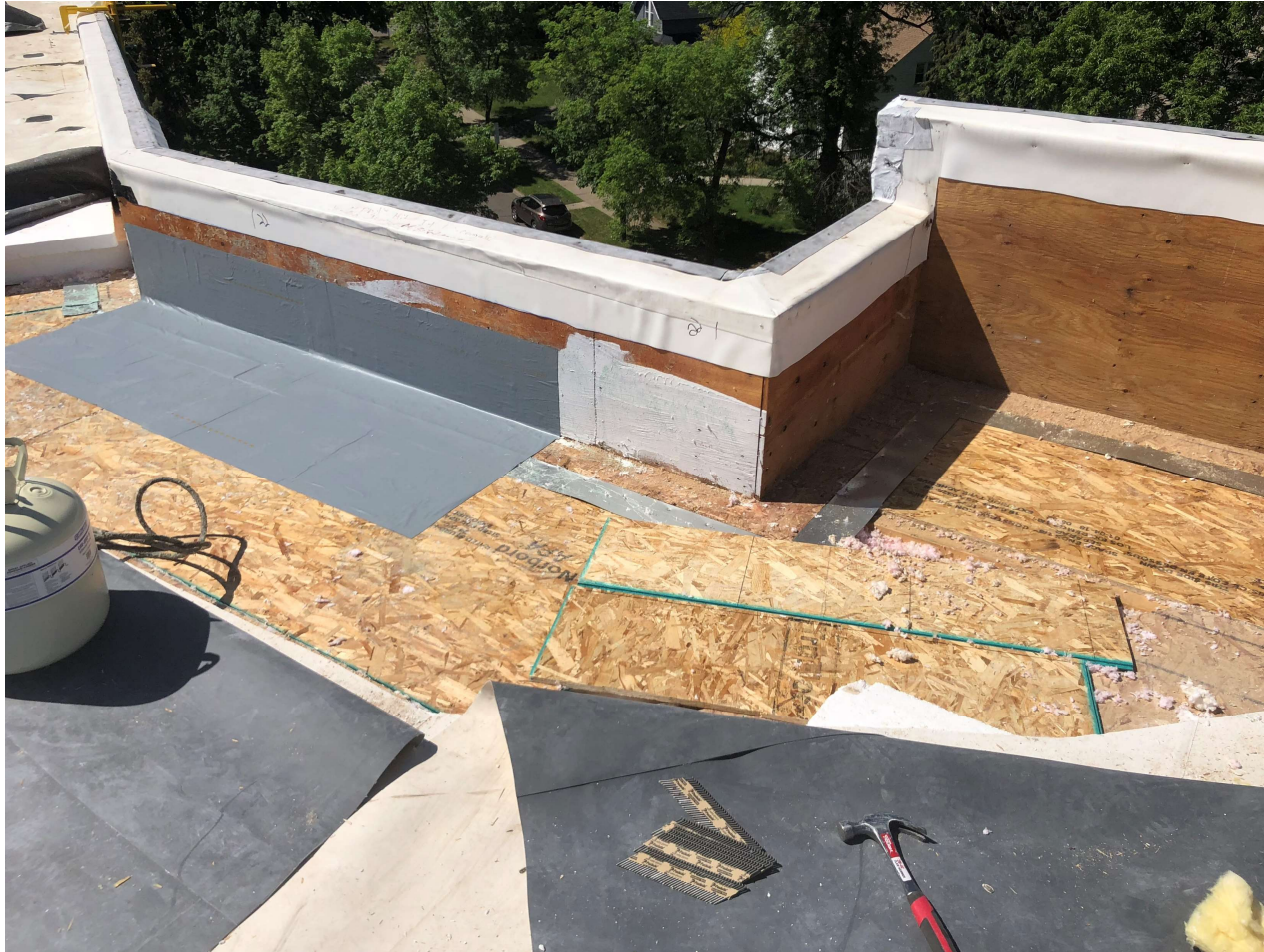
Roof vapor/air barrier at roof perimeter
