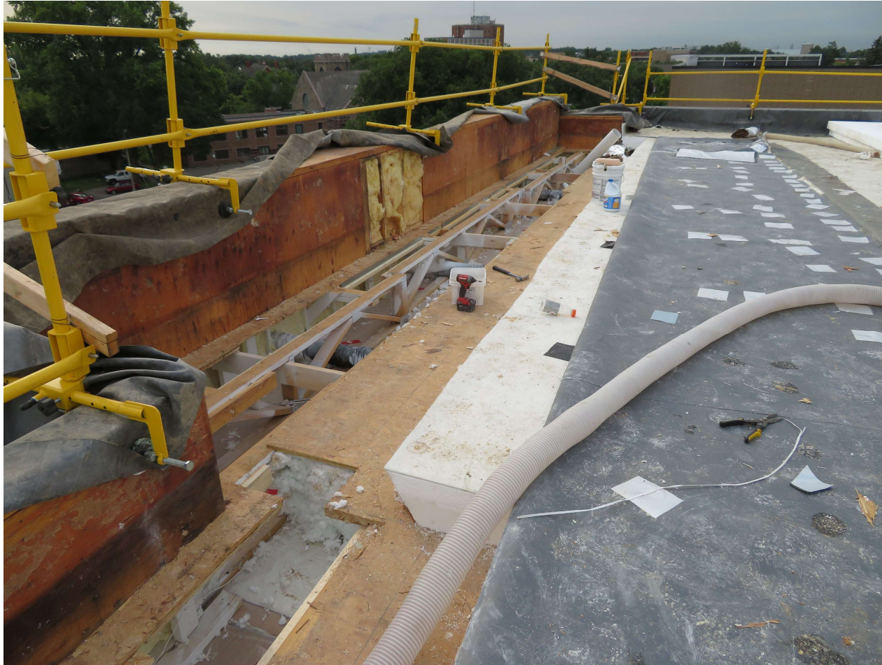
Typical work at roof perimeter
