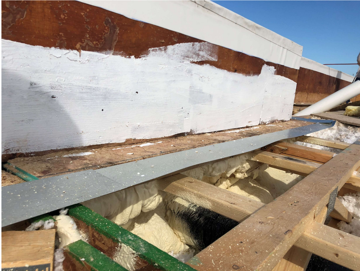
Z-shaped vapor/air barrier transition metal
